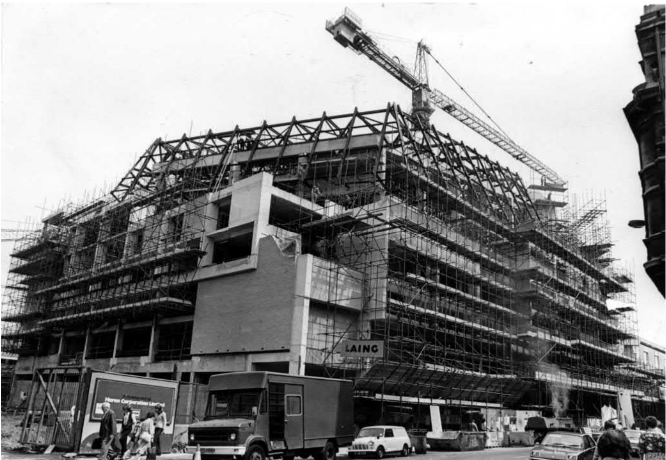
Fig.1 – St David's Hall during construction in August 1980. Source: WalesOnline
