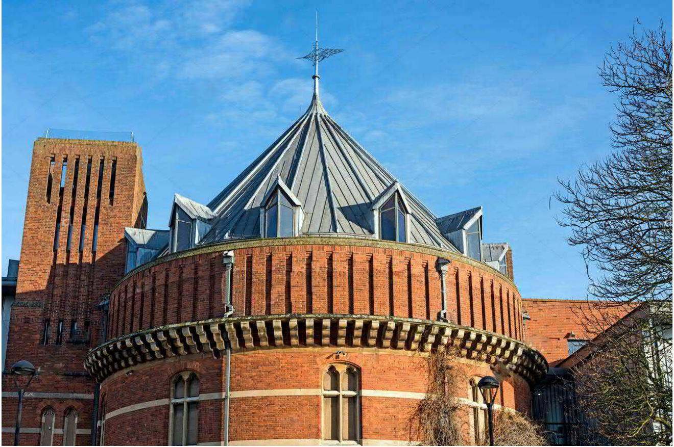
Fig.2 – Example of terne-coated steel roof covering to Swan Theatre, Stratford-upon-Avon
